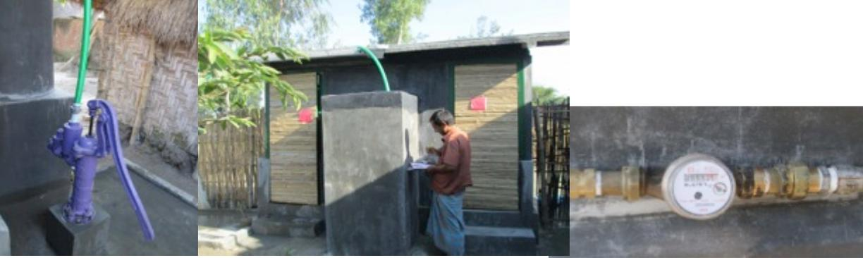
Water from rainwater and well water fills the cistern attached to the wash and toilet unit.
