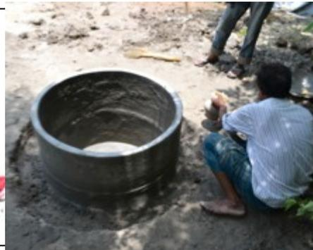
3. The redesigned waterproof construction using concrete precast rings (see details of the process)
