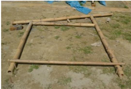
2. The bamboo frame with grout filled joints was built to assess rigidity of joints and ease of insect meshing with flush frames. This was built quickly and accurately by the teams.
