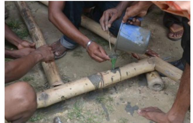
*Treated bamboo frame was assembled using grouted pinned joints (not bolts)*
